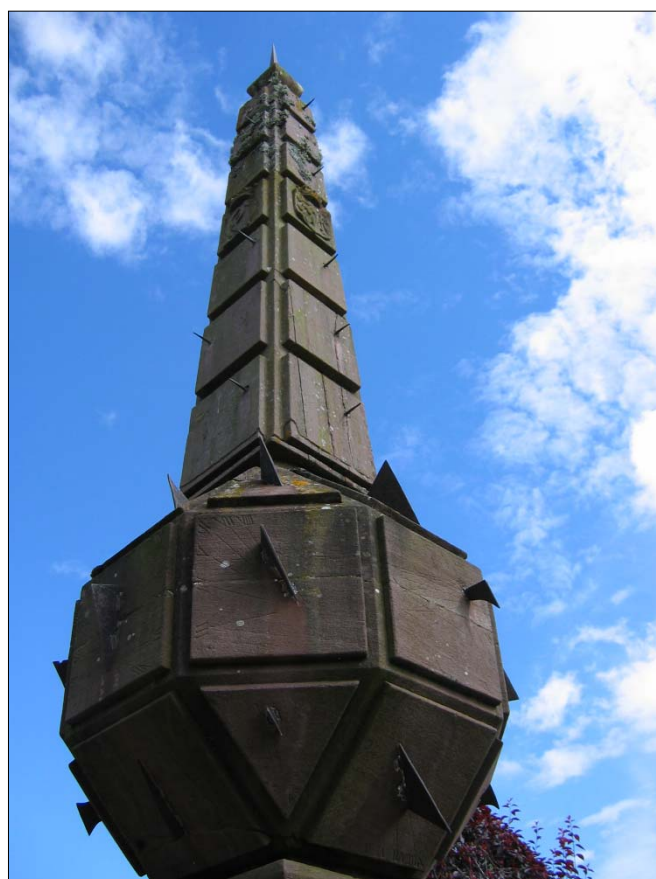
Fig. 6. The boss and finial of the Drummond Castle dial. Most of the individual dials still have their gnomons in place.
